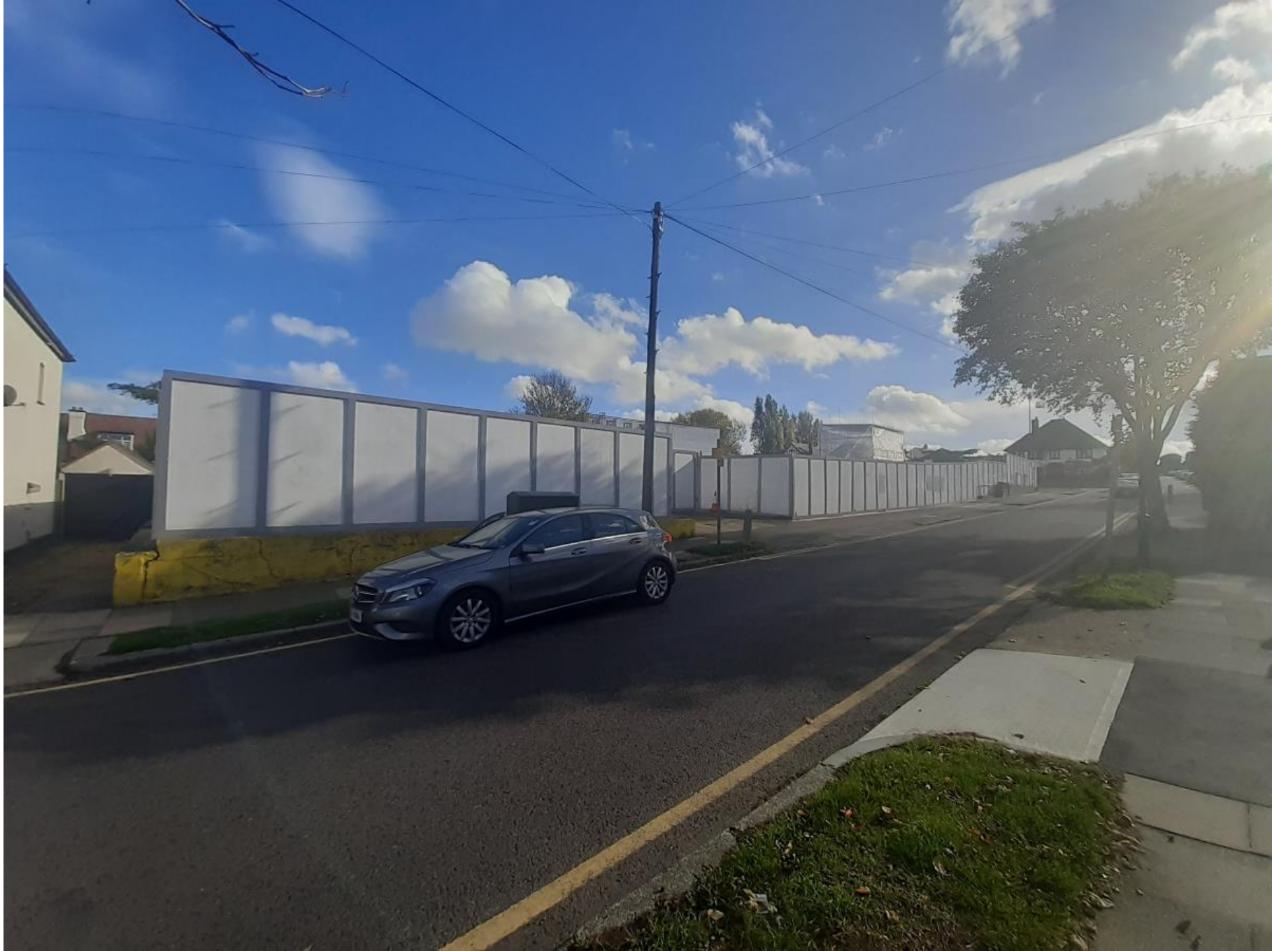
The Darlinghurst Grove frontage of the application site
